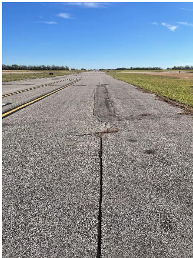
Longitudinal cracking on Runway 8-26
