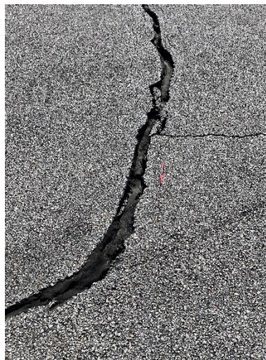
Transverse thermal cracking on Runway 8-26
